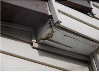
Sections of the trim need maintenance type service, and particularly on the south facing side where they are exposed to direct sunlight.
